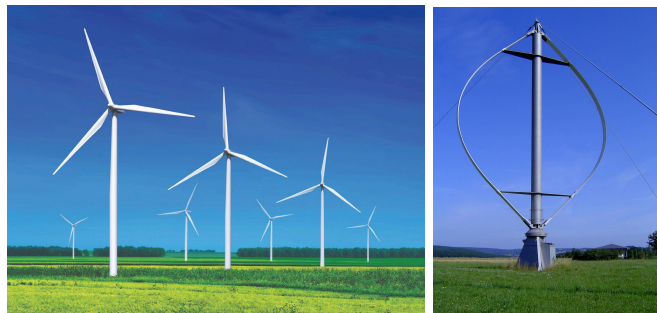
Figure 3 & 4: HAWT Wind Farm (left), VAWT turbine (right)
